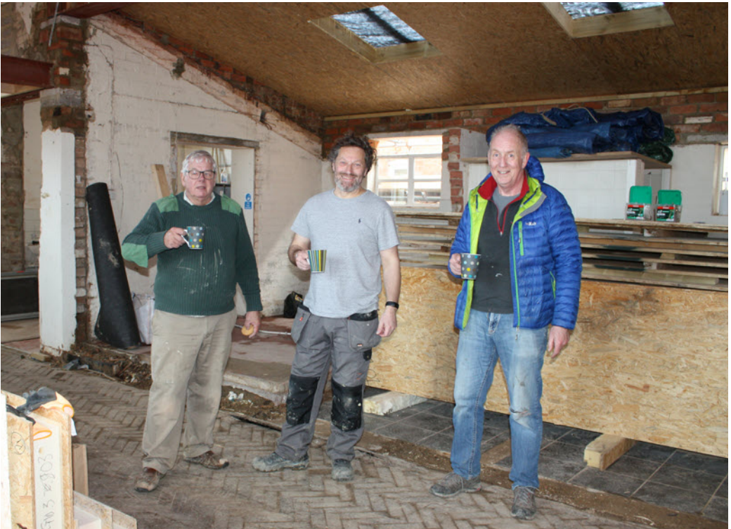
Work on the Village Hall continues at pace.
